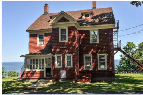
During World War II, FBI agents and radio technicians lived and worked undercover at Benson House, secretly transmitting coded messages that the Nazis believed came from their own spies. | High-res image
